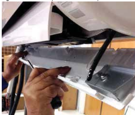
Figure 89: Remove (and Reattachment) Bottom Panel
