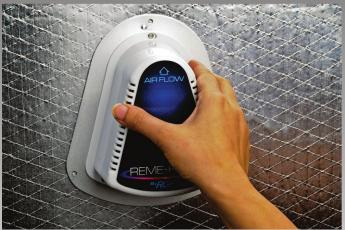
Quick Release Feature The REME HALO now features a quick release design for easy removal of the housing to allow easy replacement of the REME cell.
