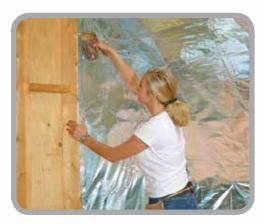
CHANNELS MOISTURE VAPOR AND ALLOWS FOR BREATHEABILITY - when vapor enters the attic from the living space, THERMO REFLECT ATTIC NT helps diffuse the vapor through its breathable membrane.
